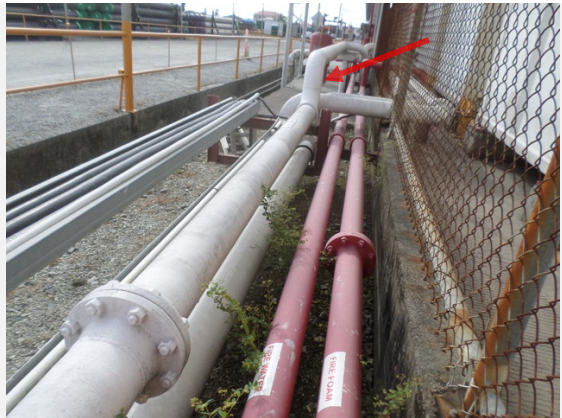
Photo: 34 Comment: General view of the line, between Pipe supports: PS52 and PS54
