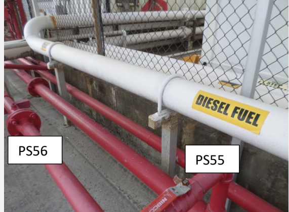
Photo: 8 Comment: Standout view of the two supports -PS55 and PS56
