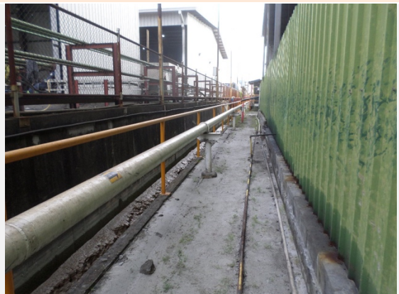
Photo: 18 Comment: General view of the line, between Pipe supports: PS23 and PS37
