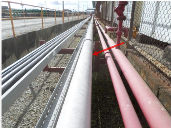
Photo: 33 Comment: General view of the line, between Pipe supports: PS45 and PS50
