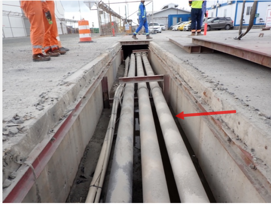
Photo: 25 Comment: General view of the line, normally located underneath the steel bridge. Good condition
