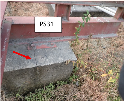
Photo: 11 Comment: PS31 – Concrete foundation – A, with crack running down the center
