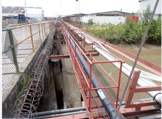
Photo: 20 Comment: General view of the wooden supports P44 – P49. Each support with two wooden pillars: A and B
