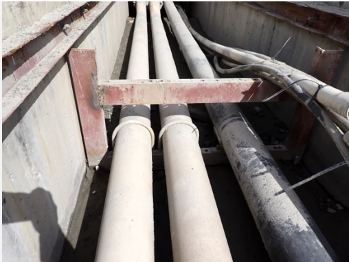
Photo: 8 Comment: Pipe support PS28 – normally located underneath the steel bridge. Surface corrosion on the support, compact soil and water present at the base.
