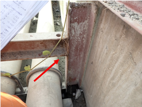
Photo: 7 Comment: Pipe support PS27 – normally located underneath the steel bridge. Surface corrosion on the support, compact soil and water present at the base.
