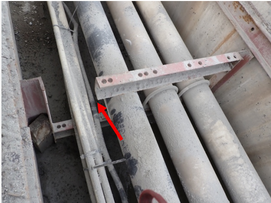
Photo: 10 Comment: Pipe support PS28 – normally located underneath the steel bridge. Surface corrosion on the support. Top bracing cut-off
