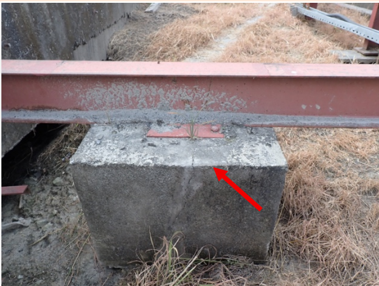
Photo: 12 Comment: PS31 – Concrete foundation- B, with crack running down the center
