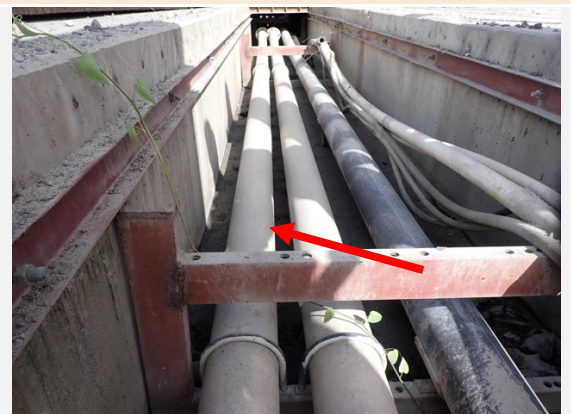
Photo: 24 Comment: General view of the line, section located between pipe supports PS18 and PS23
