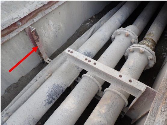
Photo: 9 Comment: Pipe support PS27 – normally located underneath the steel bridge. Surface corrosion on the support. Top bracing cut-off
