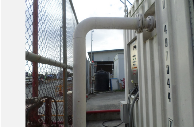
Photo: 1 Comment: View of the start of the Fuel Diesel line (Gysbi to Wharf)
