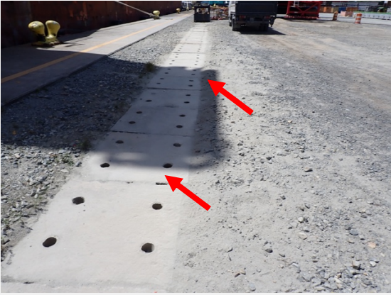
Photo: 14 Comment: Berth 3. Utilidor with the covers on. General view
