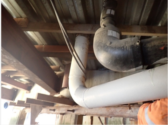
Photo: 29 Comment: Section of the line, at the penetration to berth 3, good condition
