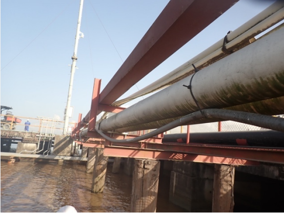
Photo: 1 Comment: General view of the Fuel line running along the bridge, into the under the wharf – good condition
