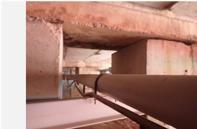
Photo: 16 Comment: General, good condition of the line, underneath Berth 2. Point 280
