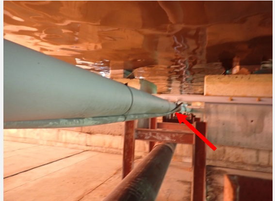
Photo: 8 Comment: General, good condition of the line, underneath Berth 1. Point 236
