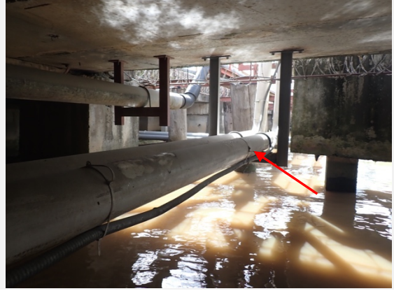
Photo:2 Comment: General view of the Fuel line running under the wharf – good condition
