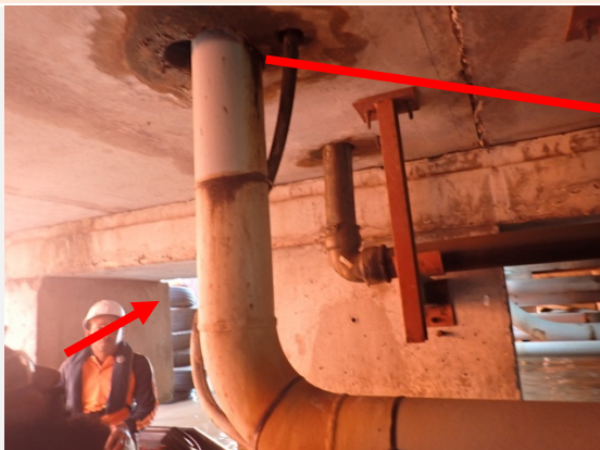
Photo: 9 Comment: Fuel line, penetration to the Manifold at the Berth 1. Point 251
