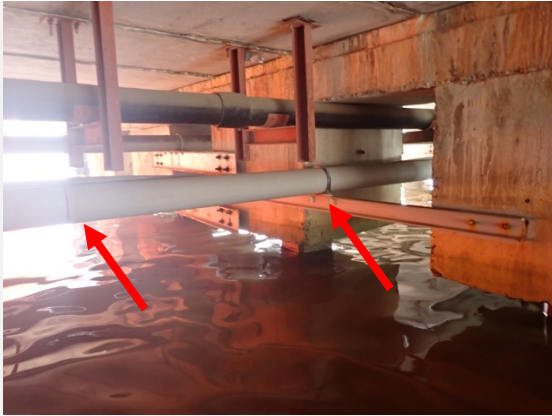
Photo: 7 Comment: General, good condition of the line, underneath Berth 1. Point 224
