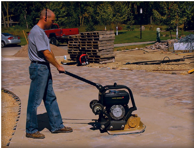
Figure 11. Vibrating sand into the joints.
