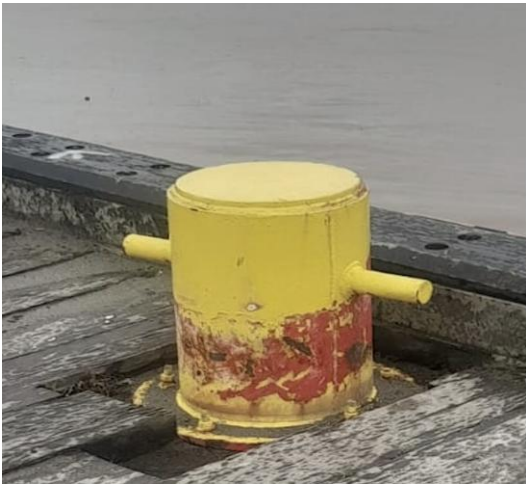
Figure 1 - Typical 15T mooring bollard
