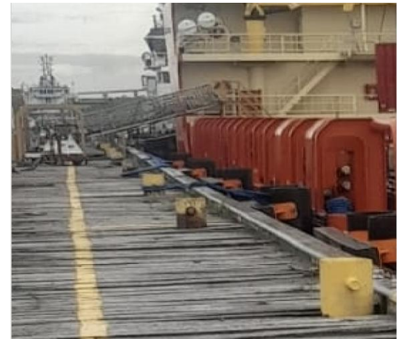
Figure 2 - Typical 15T bollard location
