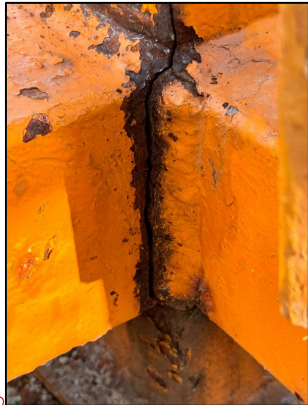
SELECTION OF EXISTING STAIR PHOTOS SHOWING EARLY ONSET AND CURRENT STATE OF CORROSION AFTER 2 YEARS SERVICE
