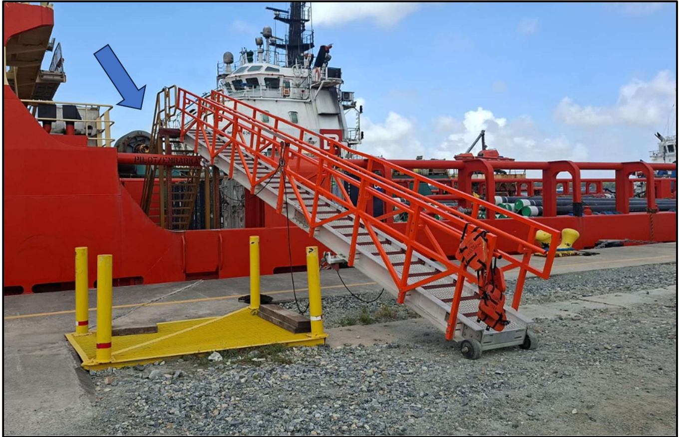
GANTRY CRANE FROM BERTH TO STAIR ASSEMBLY, TO BE REPLACED
