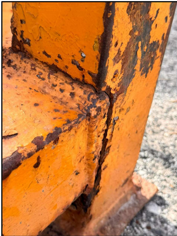
SELECTION OF EXISTING STAIR PHOTOS SHOWING EARLY ONSET AND CURRENT STATE OF CORROSION AFTER 2 YEARS SERVICE
