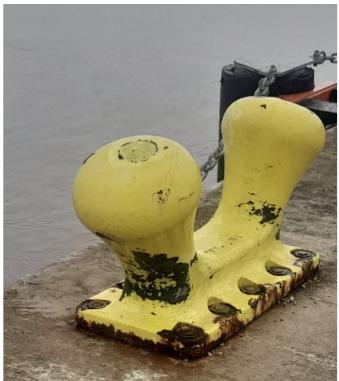
Figure 3 - Typical 50T bollard
