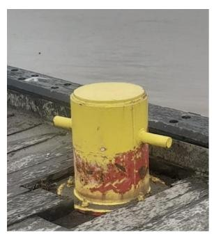
Figure 1- Typical 15T bollard
