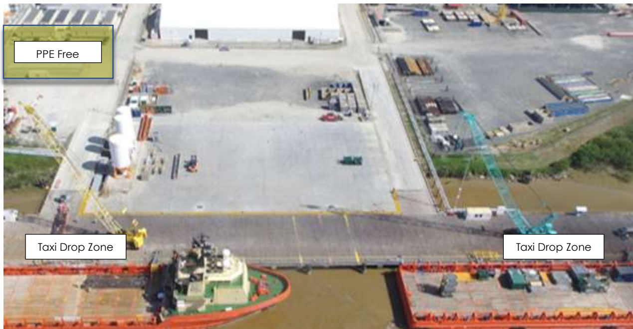
Figure 1 : Picture showing the PPE free zone and the taxi drop zone.
